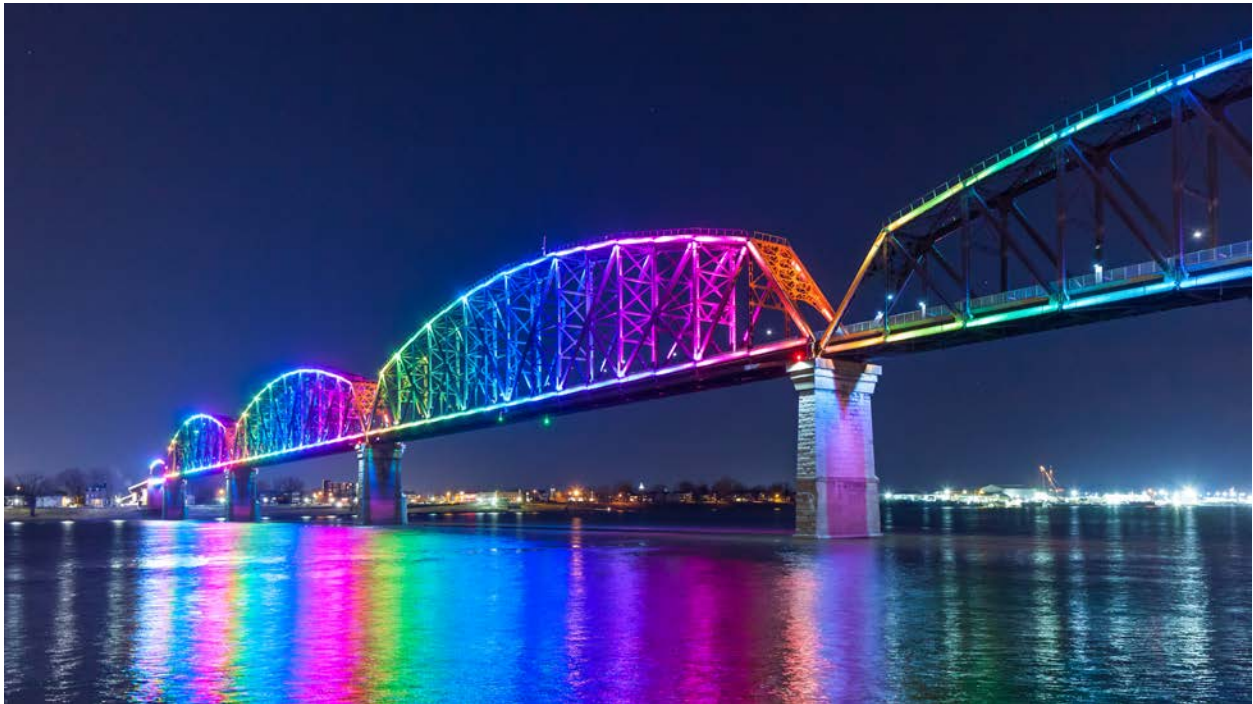
Big Four Pedestrian Bridge, Louisville, Kentucky
