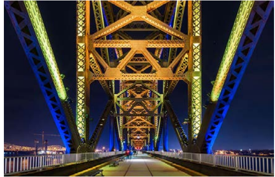
Big Four Pedestrian Bridge, Louisville, Kentucky
